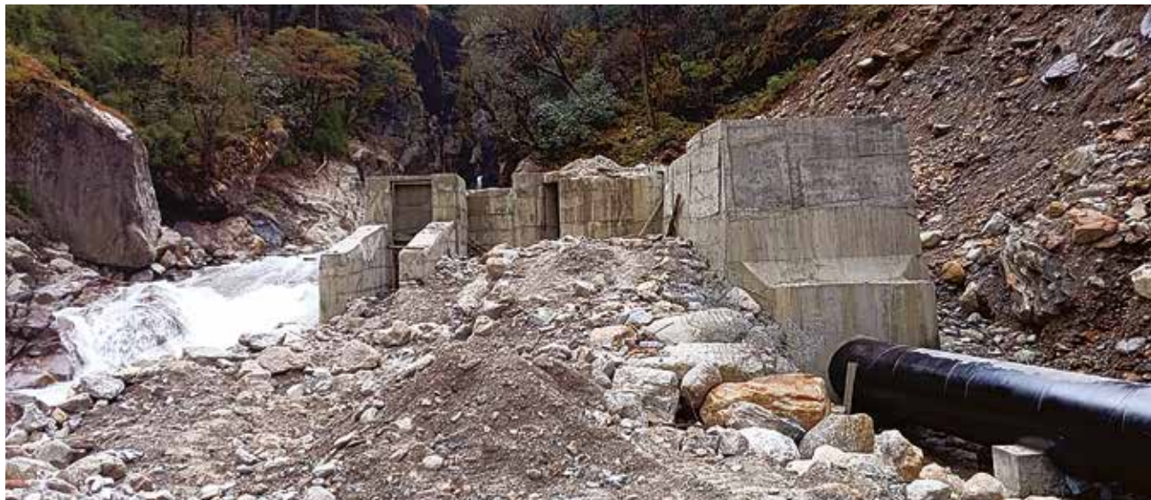
Intake and Connecting Pipe
