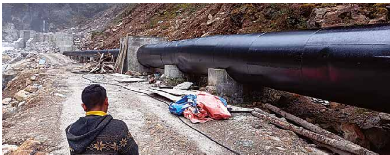
Headrace Connecting Pipe
